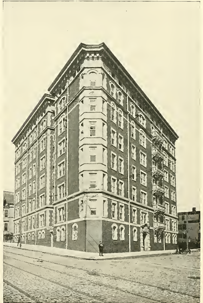
BRODERON APARTMENT HOUSE Corner High Street and Brientnall Place.
